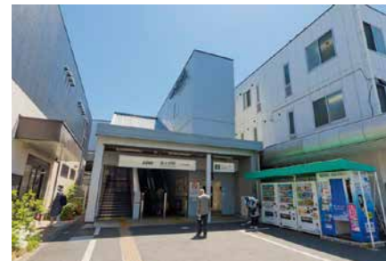
Sakurajosui station Photo by https://town.mec-h.com/mh-kyodo/82
